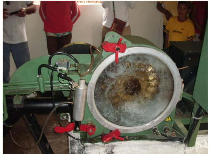
**Photo 2. Examining the Pelton wheel generator.**
