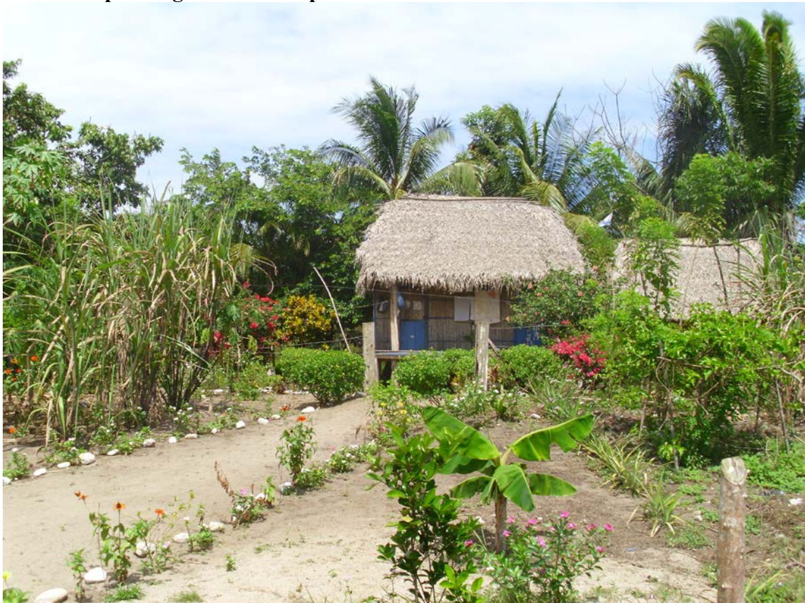
A typical grass hut, with everything tied together. No nails used
