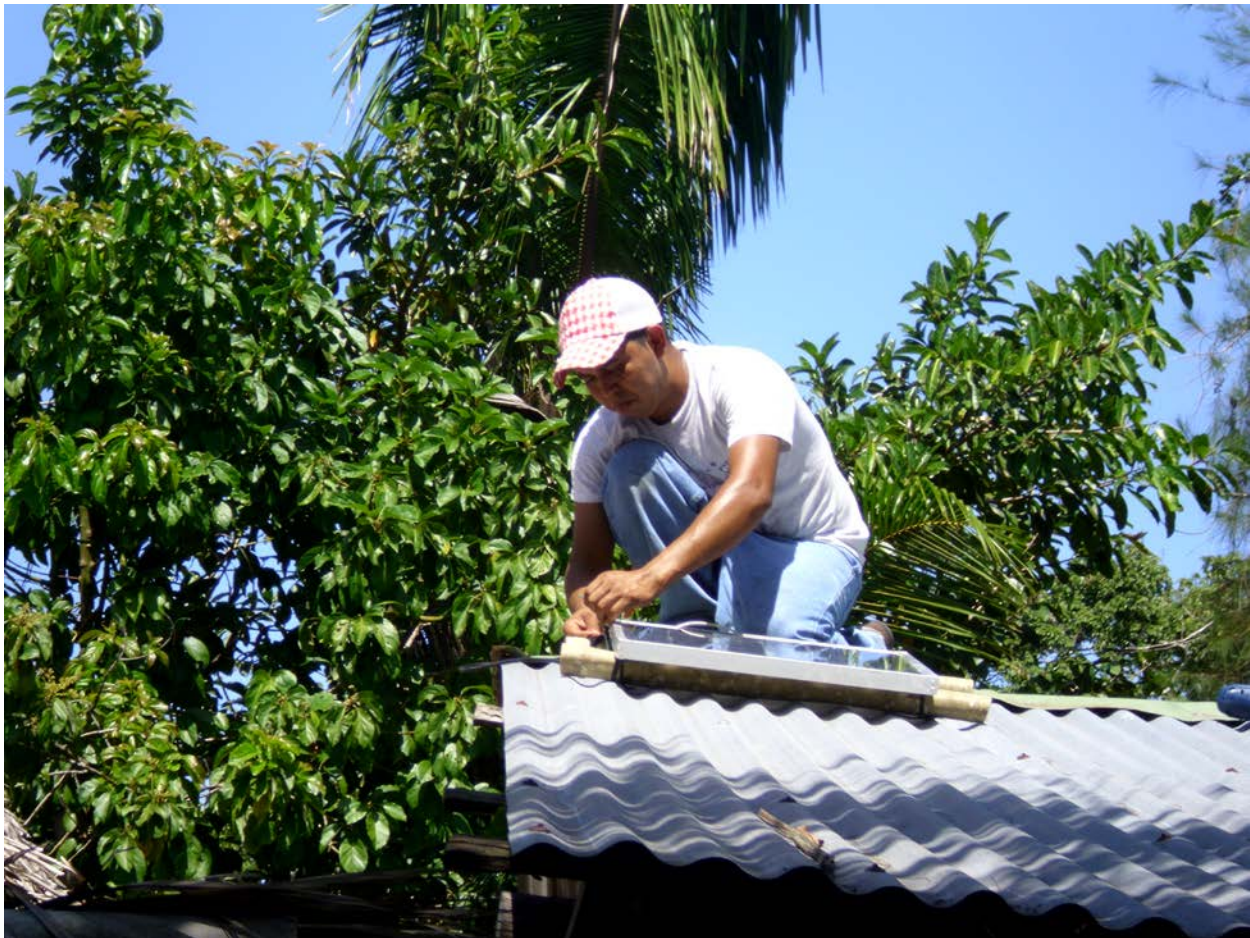
Installing the first PV system on a cottage.
